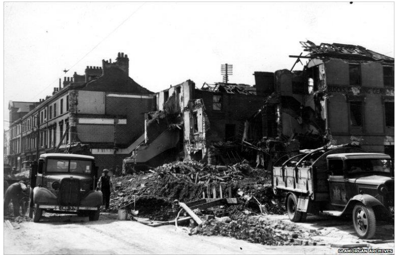
Above: Damage to the houses and bakery in Stockland street, Riverside.
